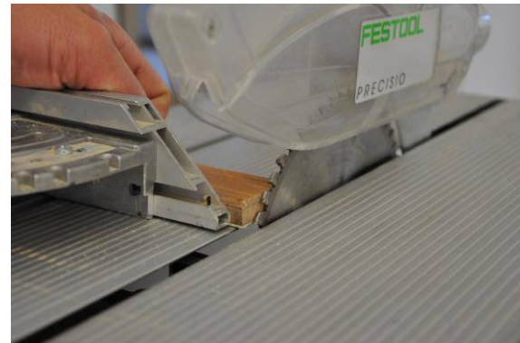
Make a 45° mitre cut in the panel at the corner of the stair nosing.
