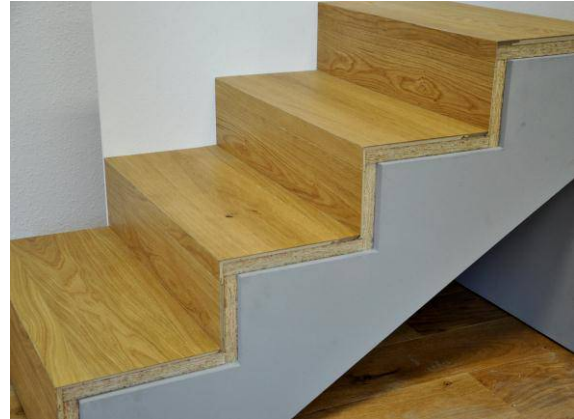
Only when the entire staircase has been glued is the outer panel cut and adjusted.
