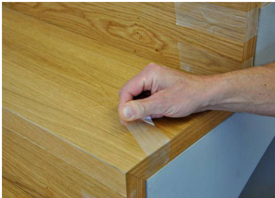
Adhesive strips suitable for coated wood surfaces are used to glue the individual panel pieces at the connections. The adhesive strips must be removed after approx. 10 minutes to avoid damage to the wood surface.
