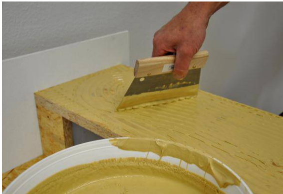
Now apply the HARO Flexible Glue to the top side of the last step shim (stair landing) using the spreader L.
