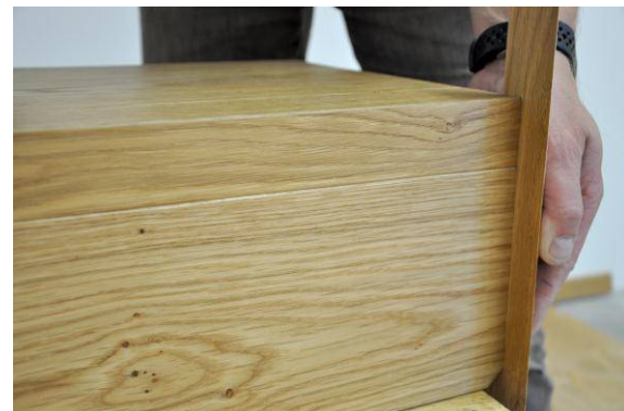
When gluing the parquet and riser boards, make sure they fit precisely at the outer mitre joint. It is recommended to place a flat surface (planed wood surface) over the outer edge of the entire mitre joint to check the precision fit of the outer mitre joint. The straight line of the connection can be checked in this way.
