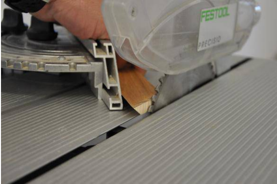
Now cut the panel to length.
